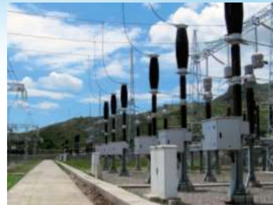
TS ELBASAN 1 220/110/35 kV Albanija
